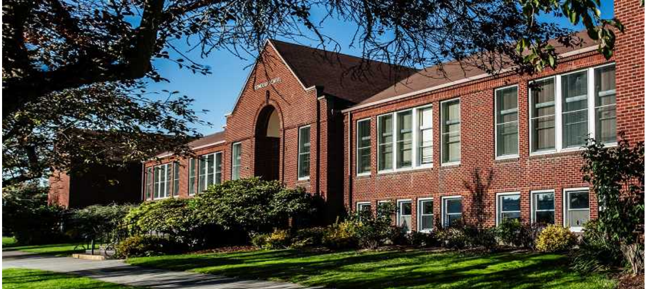
COURTESY PHOTO - Clackamas County officials are eyeing the former Concord School in Oak Grove as a site for a new library and park.
