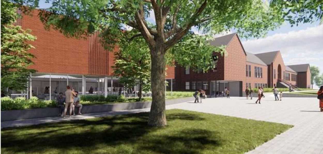
RENDERING COURTESY: CLACKAMAS COUNTY - A new Oak Lodge Library wing is proposed to be constructed next to a renovation of the current 1936 building on NCPRD's Concord School property.
